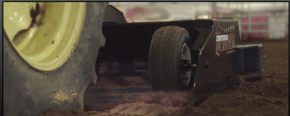
The first levelling bar creates a smooth tire path.
