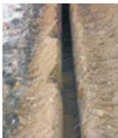
Spoil Auger moves material to one side of the trench and away from trench opening
